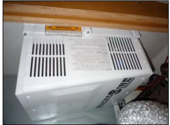
Inverter/battery charger
