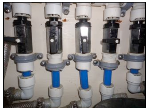
Freshwater manifold
